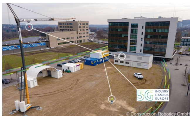
Fig. 2. Reference Construction Site, conneted to 5G-Industry Campus Europe (5G-ICE).
